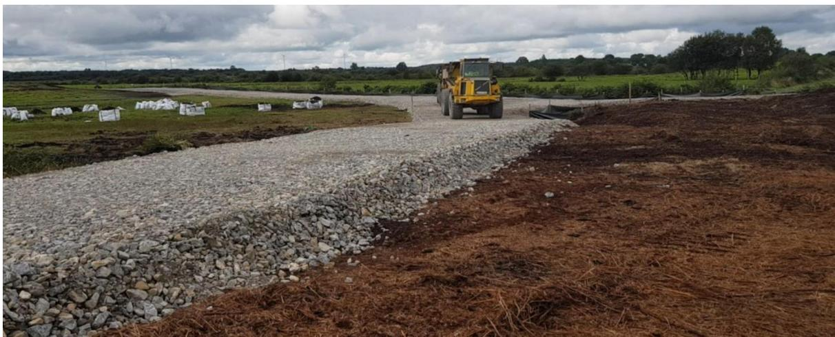
Figure 4 – Road built on existing surface without dirty water drains (2)
