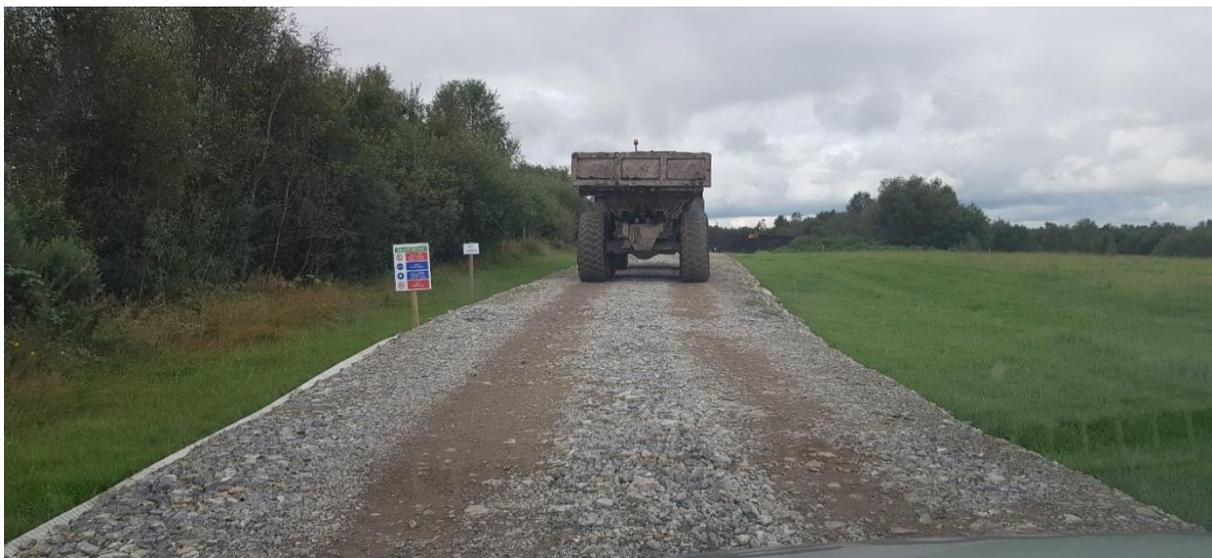
Figure 3 – Road built on existing surface without dirty water drains (1)
