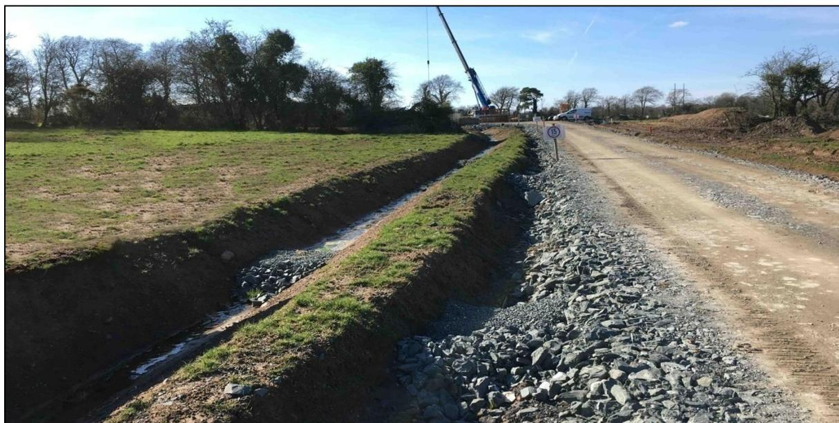
Figure 2 – Separation of clean and dirty water drainage on wind farm site
